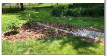
After a storm, the rain garden at the bottom of the swale (shown below) holds and absorbs runoff.
